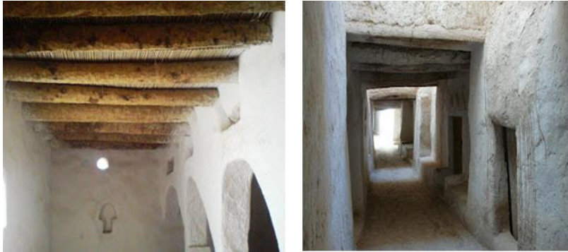
Fig3 Using palm trunks in ceiling, Source: [10].
