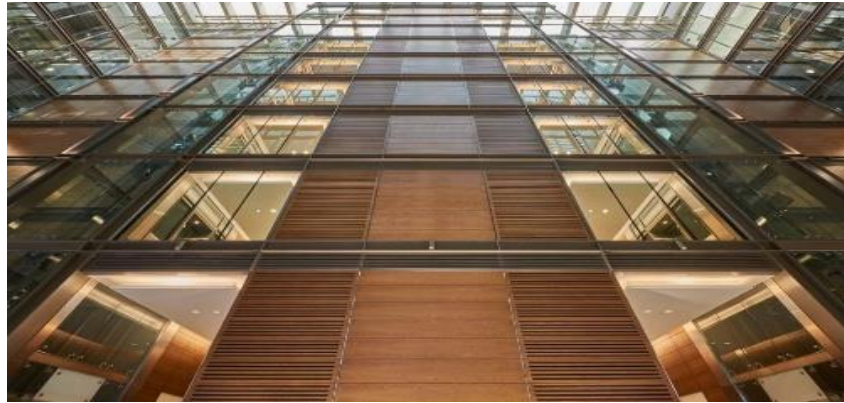
Figure 4. An interior view in central Dubai world trade Centre [11].
