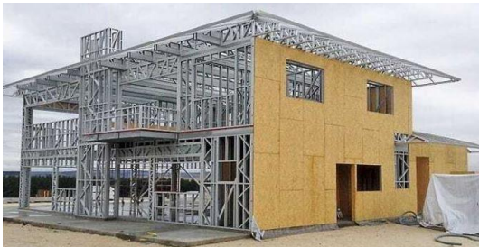
Fig. 5. Lightweight metal structures. (Obinna, 2022)
