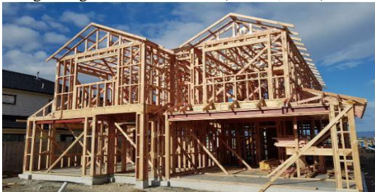
Fig. 6. Lightweight wood structures (Welch, 2022)
