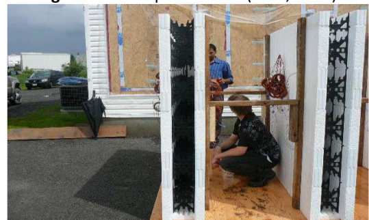
Fig. 8. Insulated Concrete Formwork (ICF) (W. Maref, 2012)
