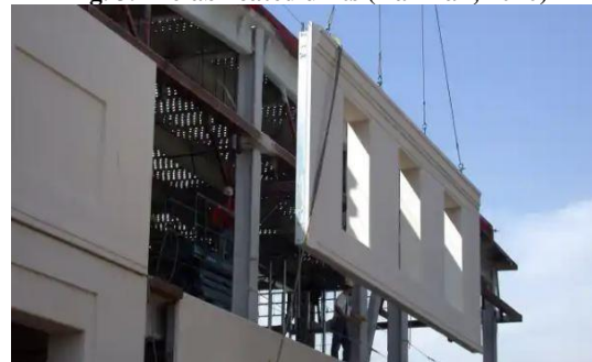
Fig. 4. . Prefabricated linear walls (Mishra, 2020)
