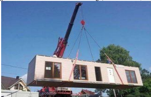
Fig. 2. Single floor Container building (Obinna, 2022)
