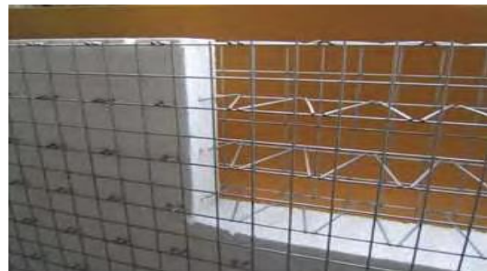
Fig. 7. EPS core panel detail (CBRI, 2017)
