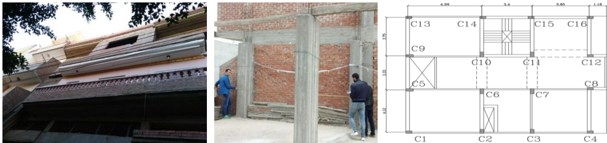
Fig 10 Building (II) Photo during field study and showing its floor structural system
