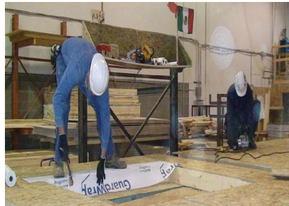
(b): window Installation carpentry crew
