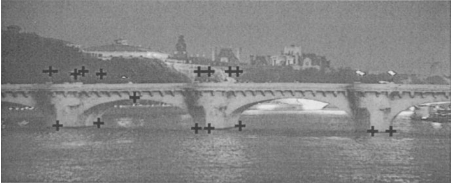
Figure 16.1 (a) The complete wire-frame model and the 3D points used for registration. (b) The corresponding 2D points extracted in an image.
