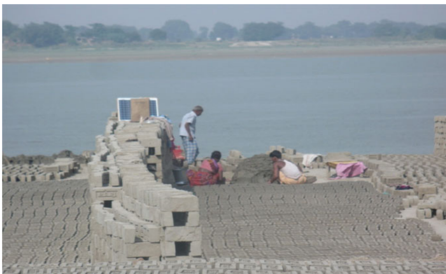
Photo 5.8 A river side brick kiln at Danapur
