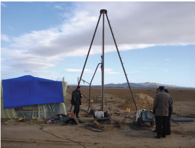
Fig. 4.14 Illegal drilling, 120 m depth with a homemade rig; Bled Sisseb north of Kairouan, 21/01/2013. The number of unauthorized wells drilled in this area is estimated to more than five hundred, and the water table has dropped by 40 m in 30 years
