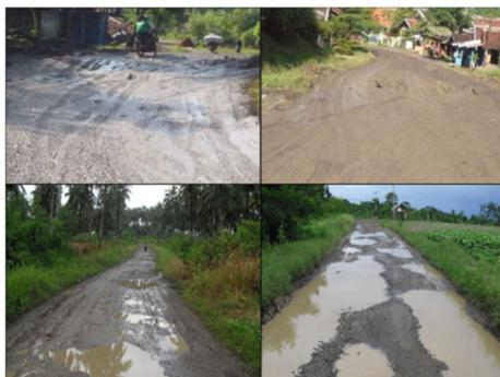
Figure 2. The condition of existing roads in the southern part of West Java before hardening with CTB.
