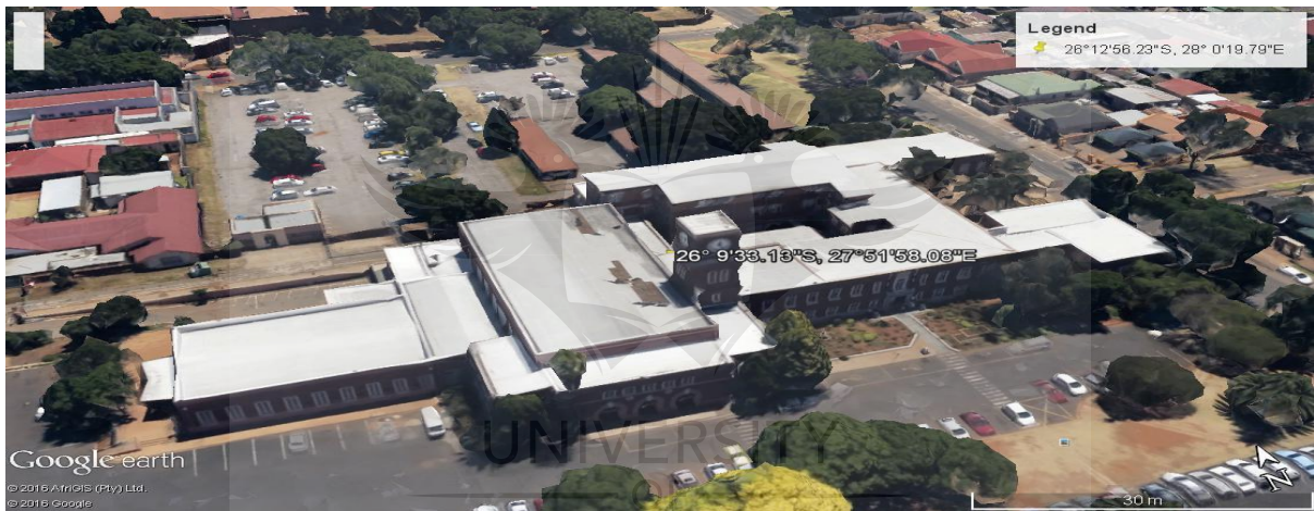
Figure 3.2: Roodepoort roof space from GEP
