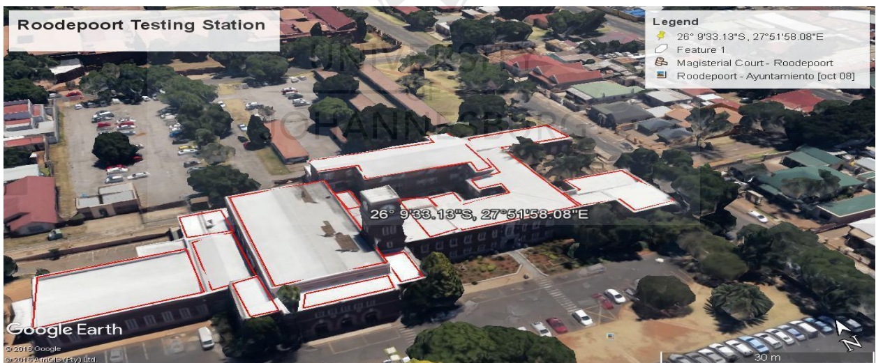
Figure 4.18: Roodepoort roof area for PV installations
