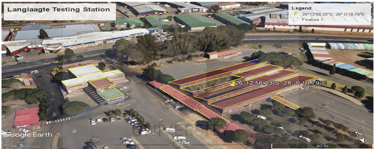
JOHANNESBURG Figure 4.6: Langlaagte roof area for PV installations
