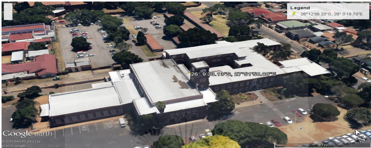
Figure 4.17: Roodepoort roof space from GEP
