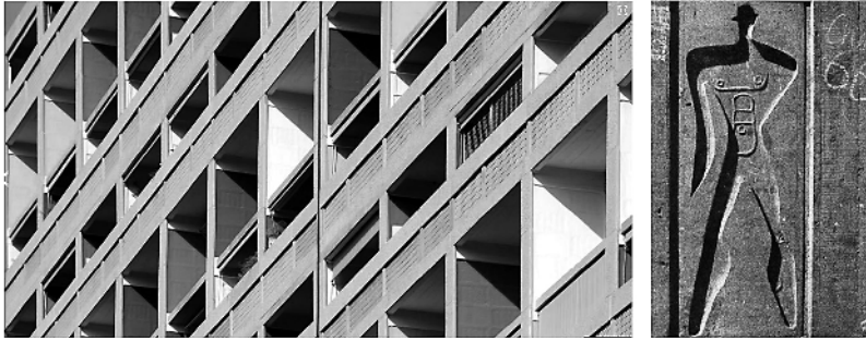
Figure 13: At Unité d'Habitation in Marseille, Le Corbusier disposed of arbitrary metric measurements and replaced them with 'the remarkable resources of numbers' derived from his Le Modulor man .
