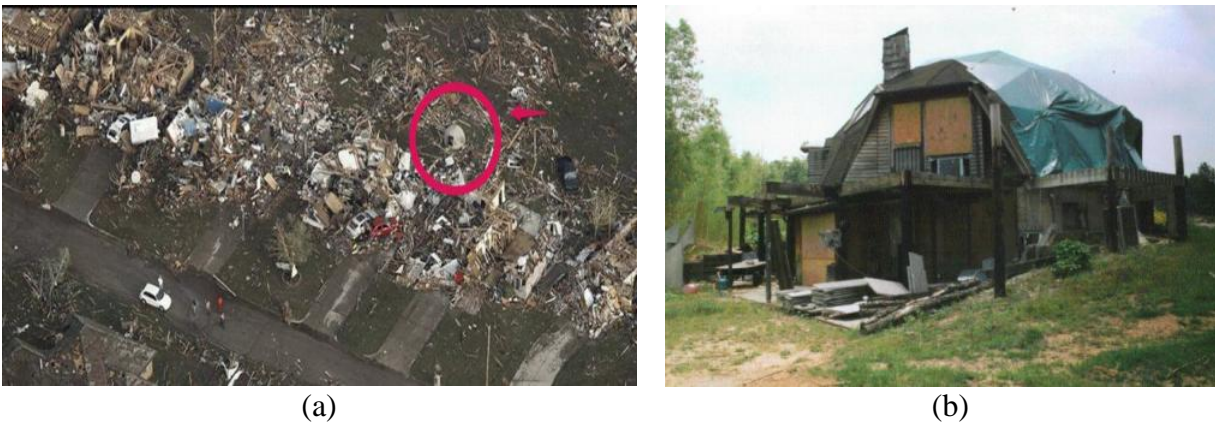
Figure 1.2: Dome survived with partial failure in (a) Moore, OK (Parker, 2011) and (b) West Jefferson County, NC (AGE dome, 2015)
