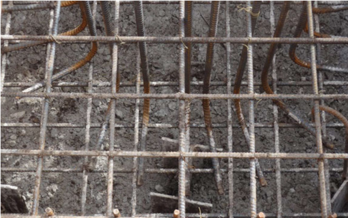
Figure 5.2 Crushed rock subbase with steel bearing pile
