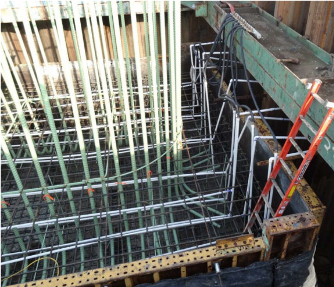
Figure 5.20 Installed PVC piping on US 34 Bridge footing
