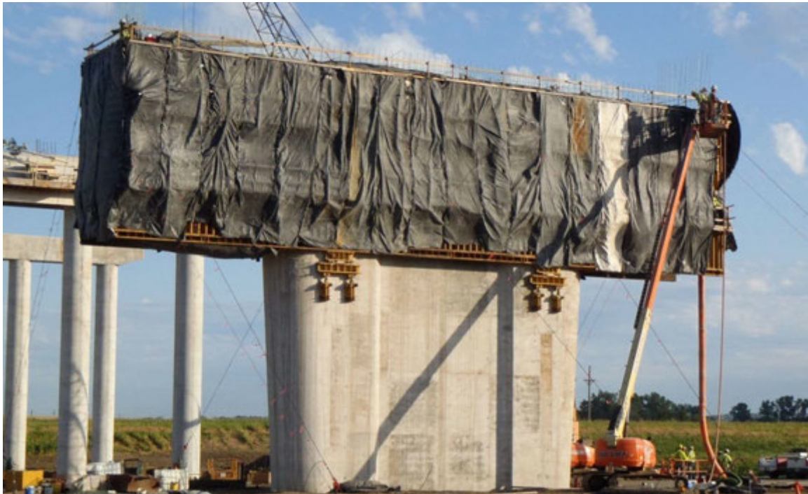
Figure 5.13 Elevated placement with insulating blankets wrapped around the catwalks
