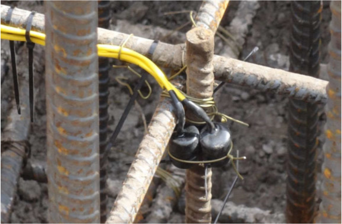
Figure A.3 Thermal sensor supported and protected with supplemental rebar
