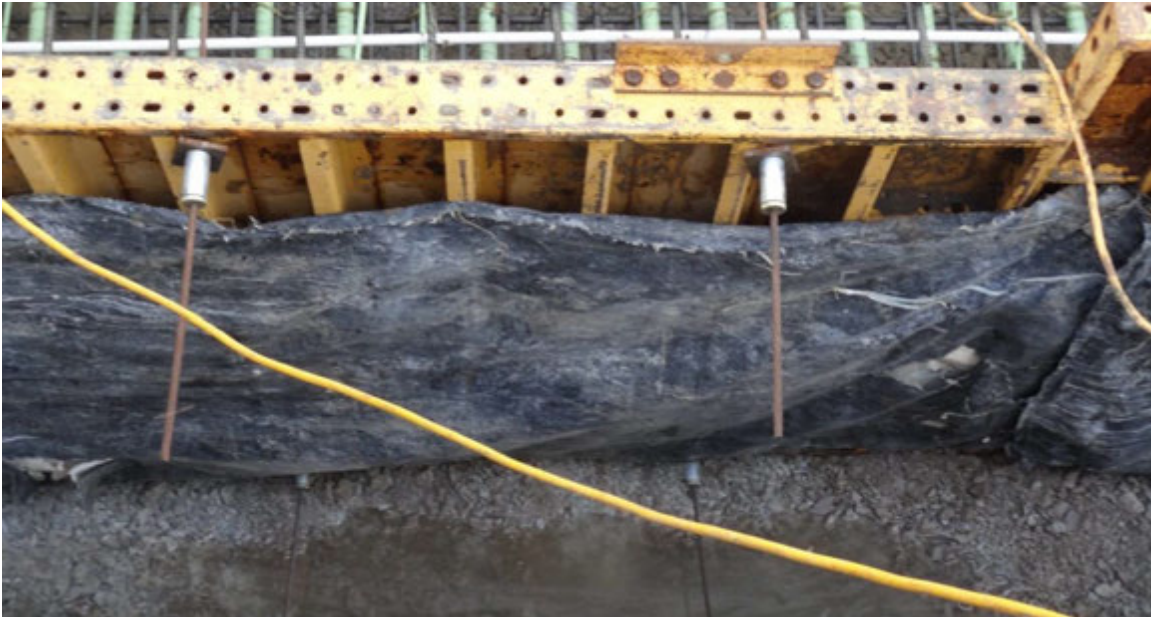
Figure 5.14 Steel formed footing with insulating blanket
