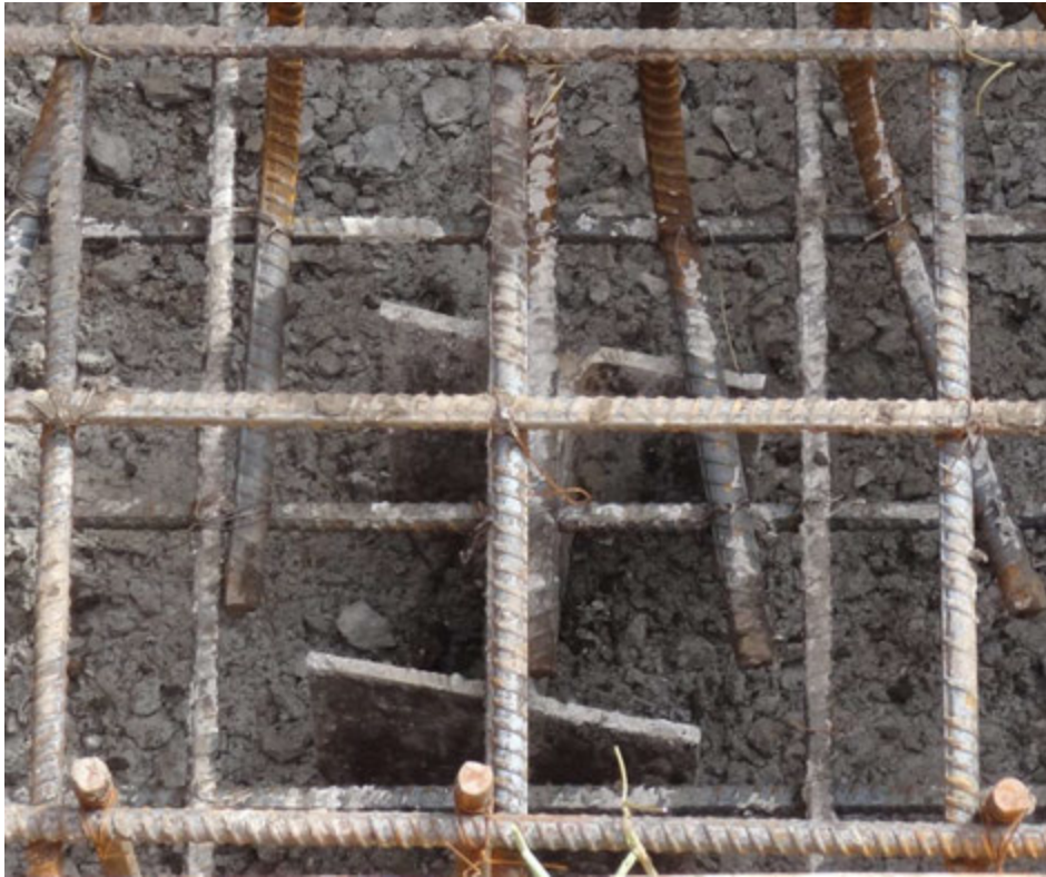
Figure 2.9 Steel pile providing external restraint to a mass concrete footing
