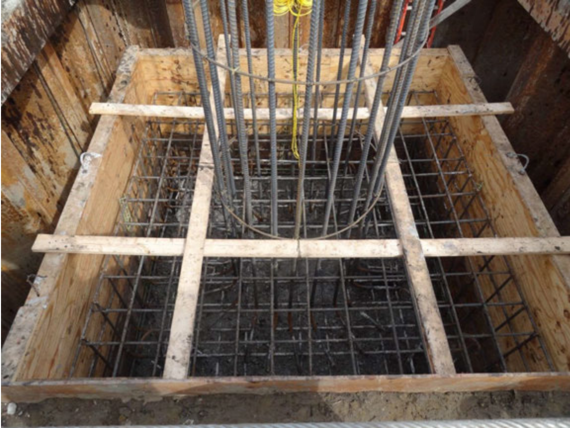
Figure 5.3 US 34 over the Missouri River Bridge Pier 3 footing
