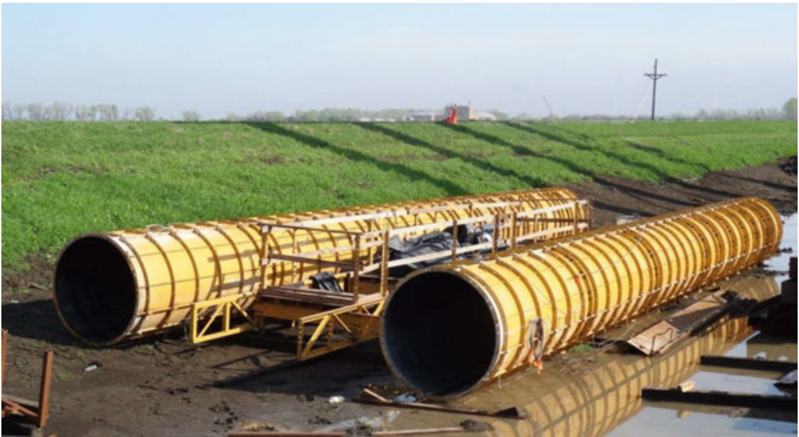
Figure 5.5 US 34 over the Missouri River Bridge column formwork
