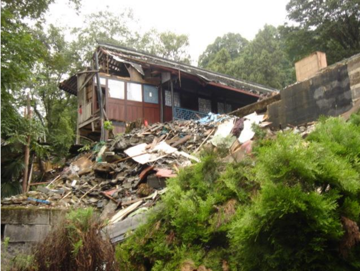
Figure 1.5. Earthquake Damage to a Local Historical Site in Dujiangyan (Source: Photo taken by Jia Lu, 2008)
