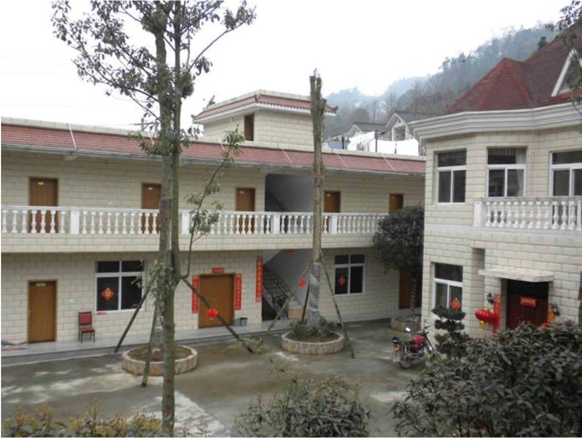
Figure A.3.8N. One Type of Joint Reconstruction with Chain Hotel Rooms and the Village Resident Housing Built Separately
