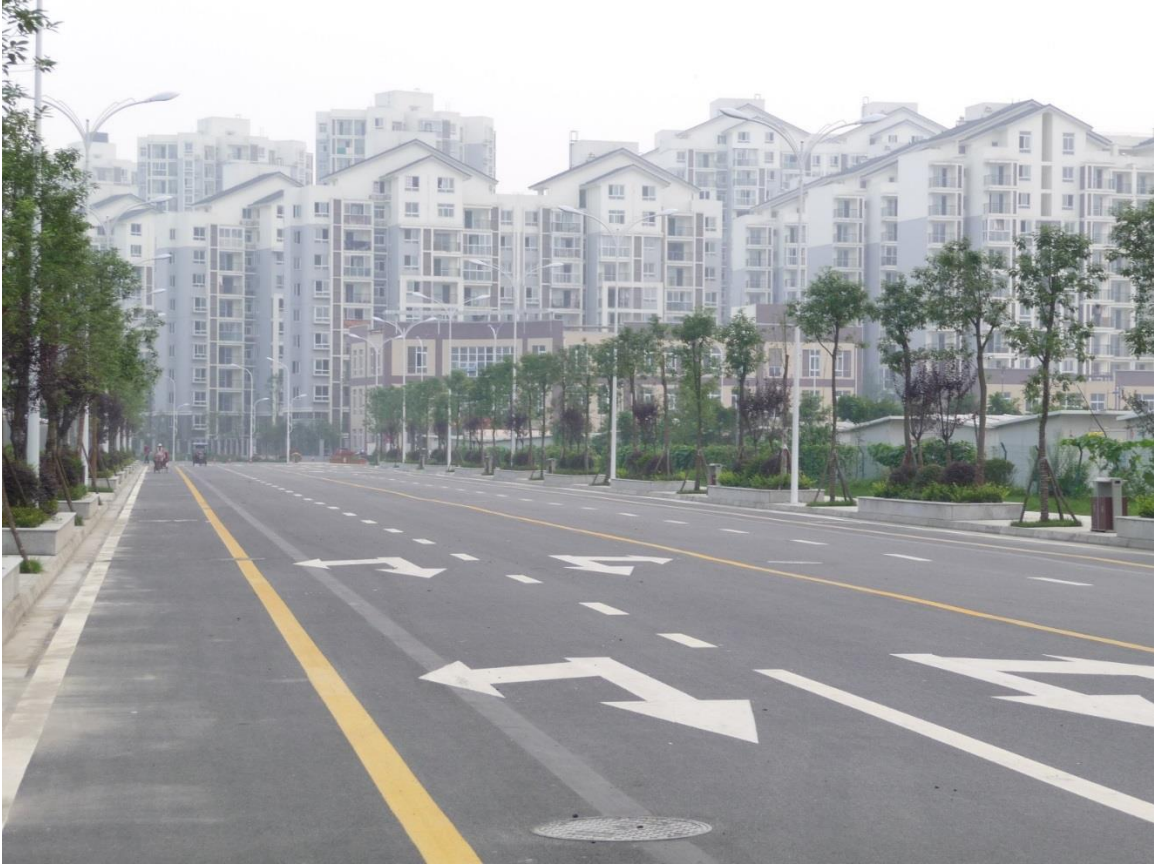
Figure 1.6. Post-earthquake Reconstructed Housing in Dujiangyan-01
