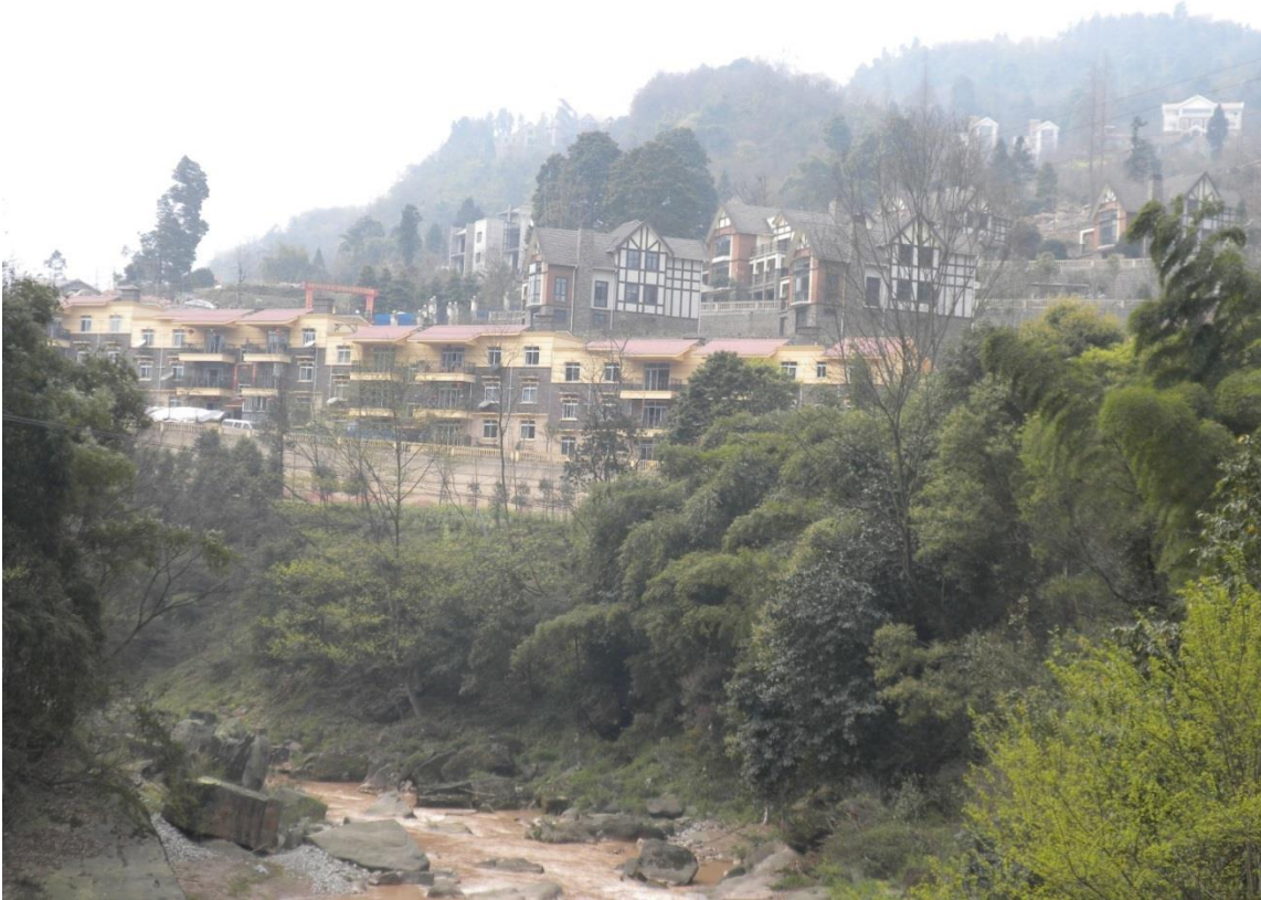
Figure A.3.8P. Partial View of the Post-Earthquake Reconstructed Housing for Local Residents
