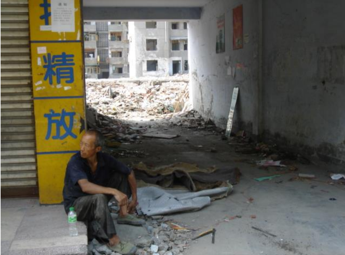
Figure 1.4. Dujiangyan Resident Sitting Outside of a Completely Destroyed Residential Site Located in the City Center Area
