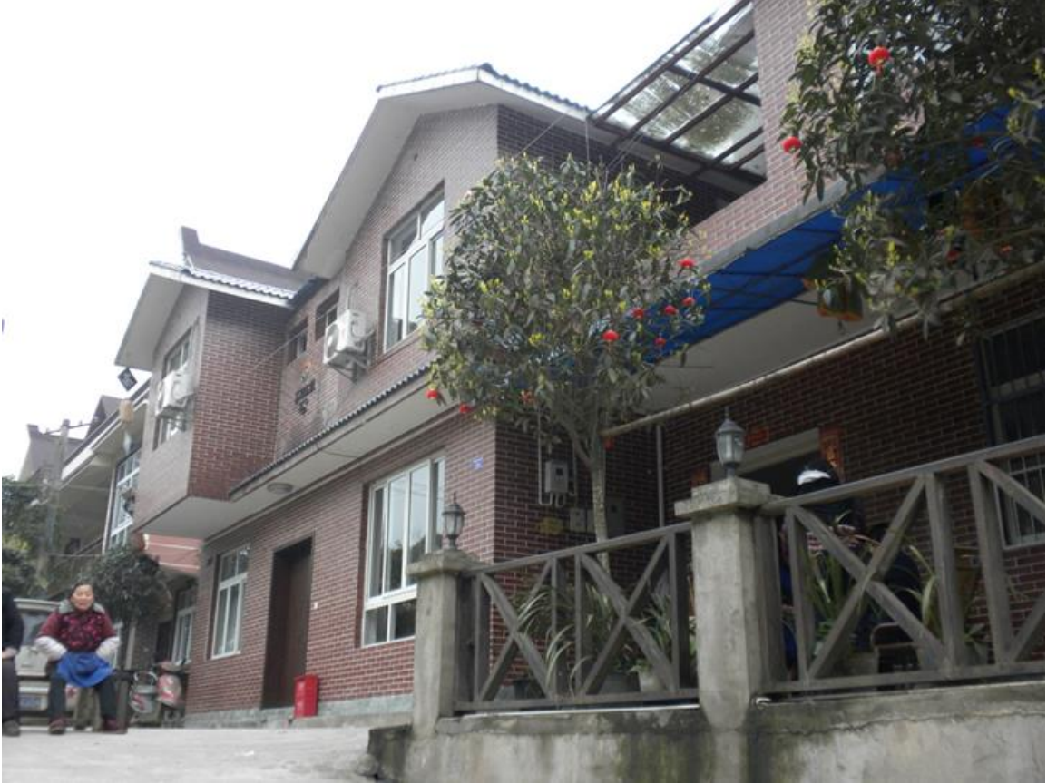
Figure A.3.8R. Residents in front of the Two-story Re-constructed Housing (Source: photo taken by Jia Lu, 2011)
