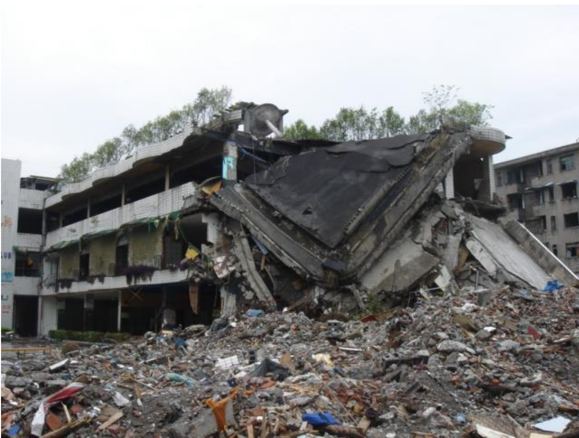
Figure 1.3. Damage of the Earthquake to a Local Hotel in Dujiangyan (Source: Photo taken by Jia Lu, 2008)
